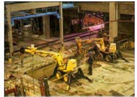
The Brokk 250 is our best selling model. It is used for many different kinds of demolition world-wide, within such industries as construction, processing, etc.
